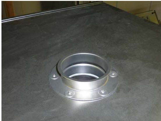
Above is with a return lip on the duct
